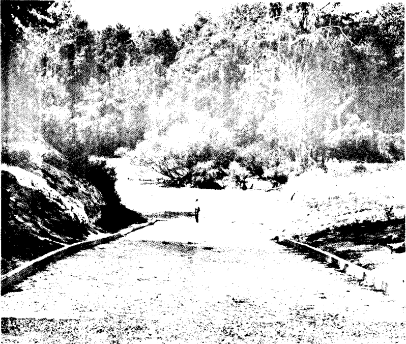
Boat ramp constructed through a deep cut in the river bank.
