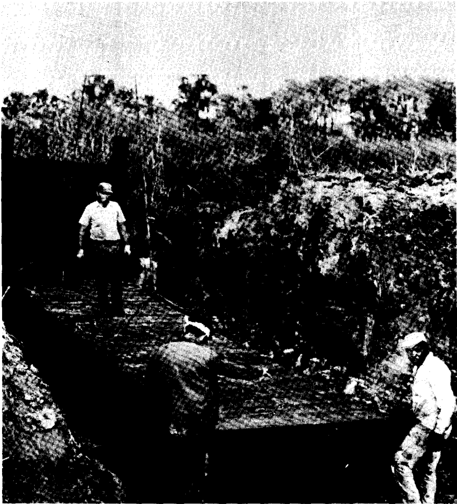
Fig. 6. Typical water control structure being installed at the Bear Island Game Management Area.
