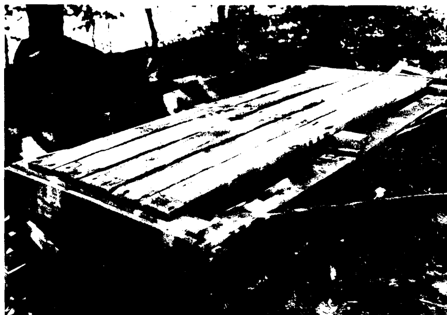
Fig. 2. 1 \times 6 's, all 8 feet long, are placed as shown for building tops. Note that nail heads indicate the 32-inch space for the five 1 \times 6 's. To build sides, seven 1 \times 6 's are placed on the 42-inch 2 \times 4 's.
