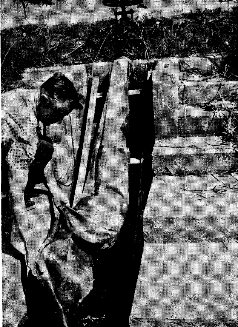
Figure 1. Saran cloth bag filter installed. Note small fish and debris collected in lower section of bag.
